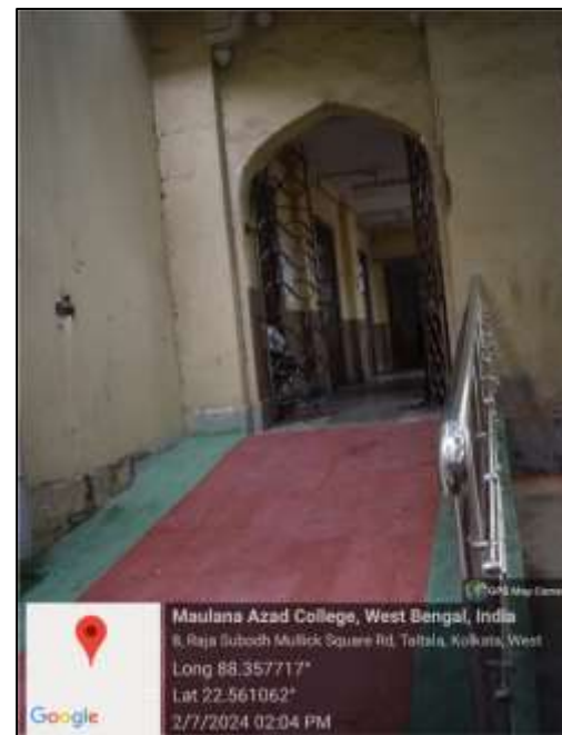
Ramp 2 with tactile path and rail leading to College Hall at ground floor
